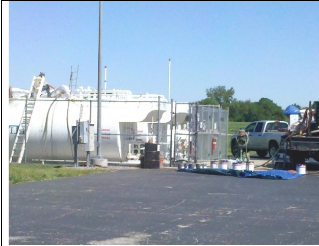
LWC 100 LL fuel tank relining
