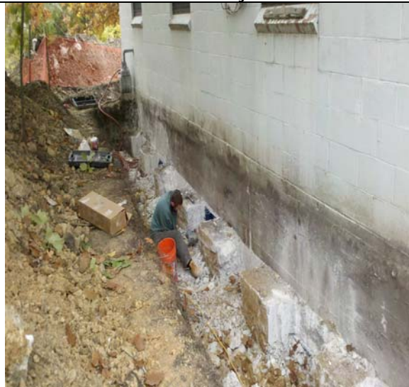
Traffic Building Stabilization
