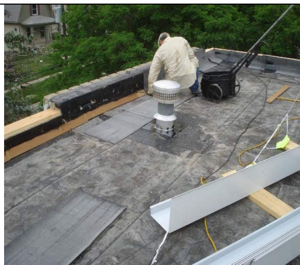
Traffic Roof replacement
