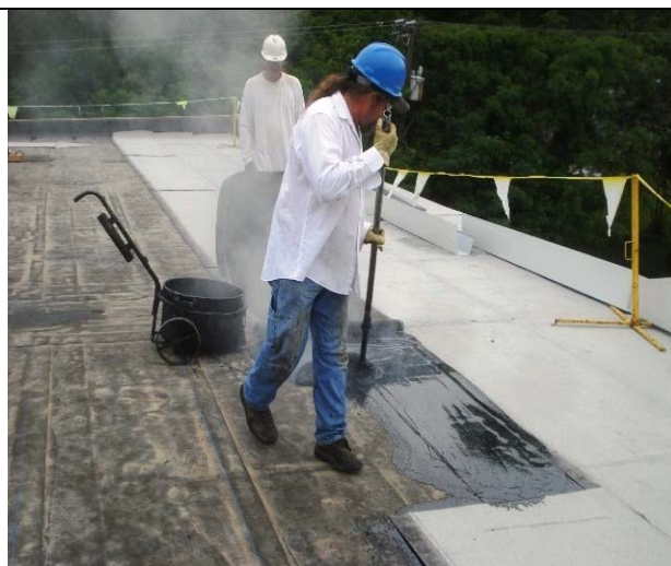
Traffic Roof replacement
