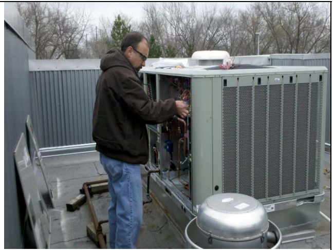
Fire/Med HVAC replacement
