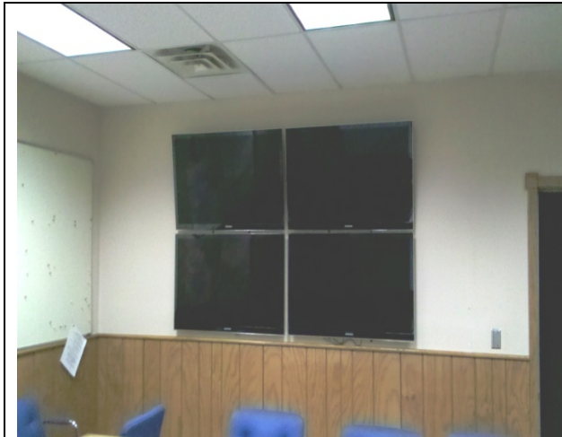
Traffic Division remodel
