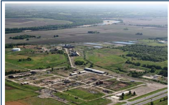
The former Farmland Industries fertilizer plant is being redeveloped for future industry.
