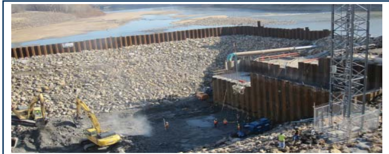
Construction crews hit bedrock during construction of the BMPC powerhouse.
