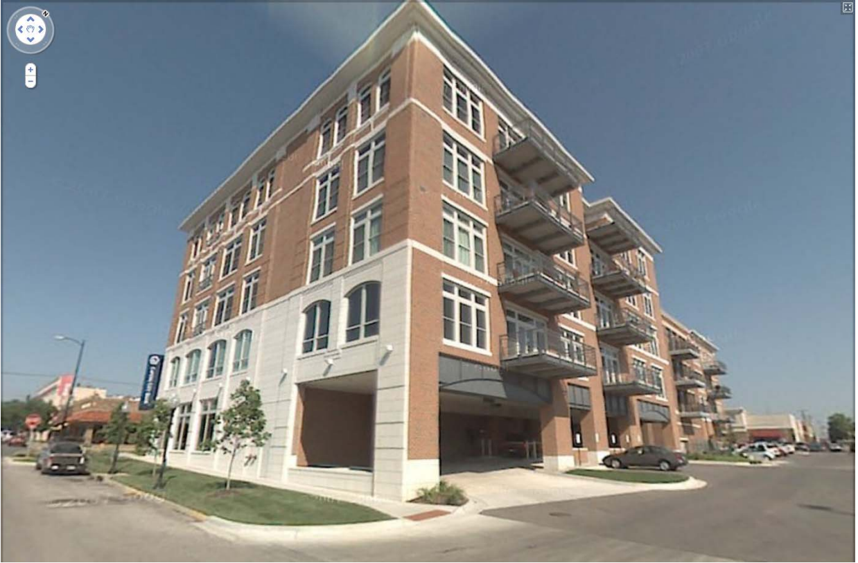
Hobbs Taylor Loft Condominiums 730 New Hampshire Street
