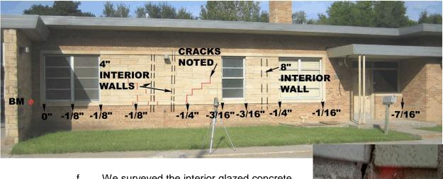
f. We surveyed the interior glazed concrete masonry unit wall mortar joints and noted cracks and settlement at some locations. A summary of the survey is on the next page. The red numbers are relative to elevations noted as "0".
