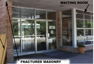
building wings). Inside this entrance we noted the brick wall was cracked at the door jamb.
