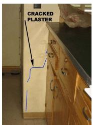
vestibule area was reviewed so the interior side of the exterior wall could be viewed. There was some cracking of the plaster finish above the entrance and along the left jamb at the corner.
