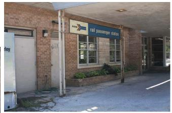
drawings. The corner of the planting bed wall is cracked and there is are several fractured brick in the rowlock cap.
