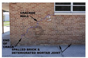
before the base of wall. There is also spalled brick and deteriorated mortar joints along the base of wall at this location.
