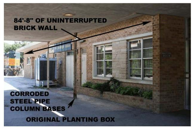
> (10) At the right end of this long wall there is a wing wall at the vestibule entrance (reference page 7). The brick wall is fractured at the beam bearing elevation. Closer examination reveals cut brick to form the beam pocket.
