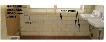
exterior wall. The crack continues into the stall next to the corner.
