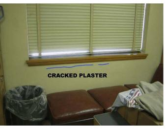
cracking of the plaster finish below and to the left of the window. The pealing paint noted suggests that moisture has been moving through the wall.
