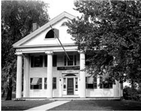
shutters. Photo: HABS collection, NPS.
