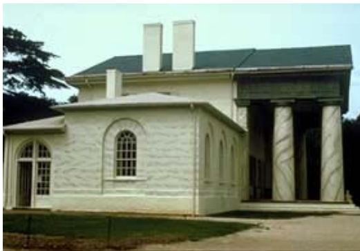
The stucco finish on Arlington House, Arlington, Virginia, was marbled in the 1850s, approximately 30 years after it was built, but because it is a character-defining finish that has gained significance over time, it should be retained and preserved. Photo: NPS files.
