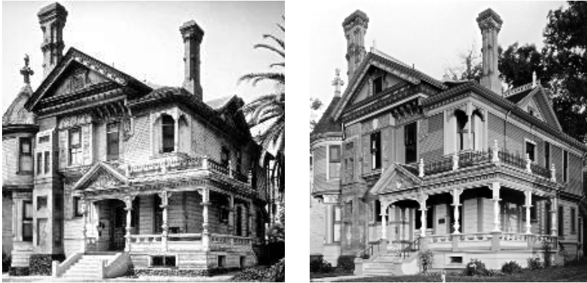
Preservation of the exterior of the Hale House, Los Angeles, California, involved repainting the exterior walls and decorative features in historically appropriate colors. In excellent example of the Preservation treatment focused upon the ongoing maintenance of historic materials and features. Photo: Before, NPS files; After: Bruce Boehner.
