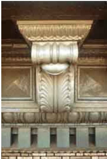
moldings after Preservation work, including repainting of the elements, has been completed. Photo: Michael Devonshire.
