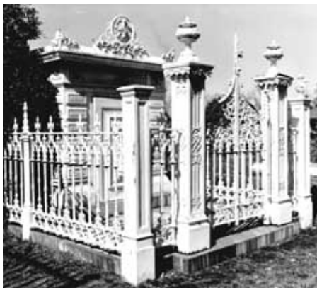
The Slatter Family Tomb in Mobile, Alabama, consisting of a cast-iron mausoleum and fence, exhibits the wide range of uses of the material in the 19th century. These historic materials should be carefully maintained and repaired. Photo: Jack E. Boucher, HABS Collection.
