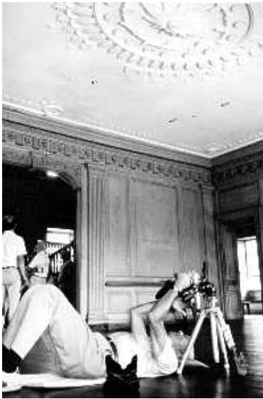
Careful documentation of a building's physical condition is the critical first step in determining an appropriate level of intervention. This may include documenting a particular problem, such as this cracked ceiling (left); or relating the historical research to existing materials and features (right). Photos: NPS files.
