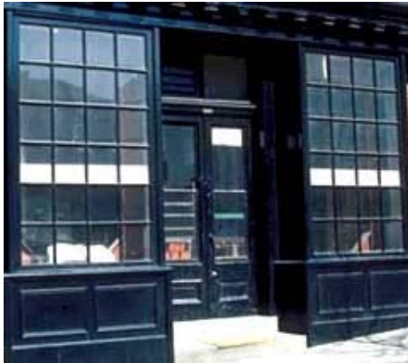
This cast iron storefront from the late 19th century has been well maintained over the years. Photo: NPS files.
