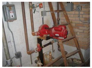
**Photo #5** View of one of three hot water circulating pumps that distribute hot water to the under floor heating system and several fan coil units.
