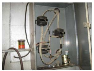
**Photo #26** View of CTs in cabinet next to meter in the boiler room.
