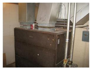
**Photo #11** View of 10 ton floor air handling unit located in the baggage area.
