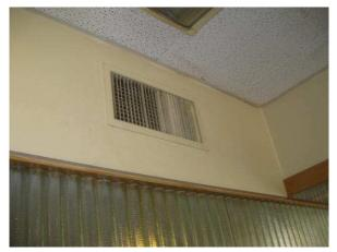
**Photo #15** View of supply air diffuser with ductwork in soffit in the main lobby of the station.
