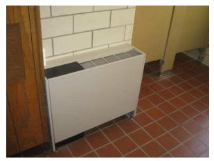
**Photo #12** View of small hot water convection unit in one of the restrooms.
