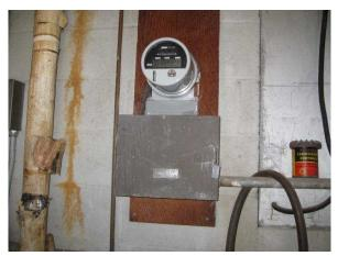
**Photo #25** View of utility meter for the 120/240 volt 3 phase high leg electrical service located in the boiler room.
