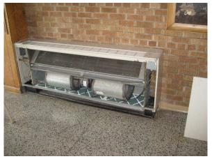
**Photo #7** View of heating only fan coil unit with front cover removed located in the main lobby of the station.
