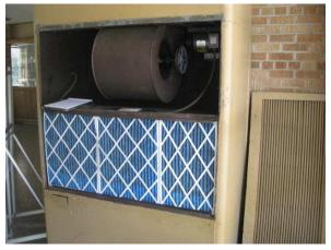
**Photo #10** View of 7.5 ton floor air handling unit located in the main lobby area.
