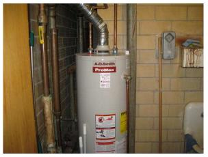
**Photo #19** View of six month old 40 gallon 40 MBH natural gas fired water heater serving the restrooms and the lavatories located in the offices.
