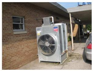
**Photo #1** View of six year old Marley cooling tower located on the platform on the north side of the station.
