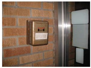
**Photo #14** View of older thermostat controlling air lock hot water convection unit.
