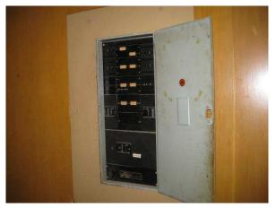
**Photo #27** View of 400 amp 120/240 volt 3 phase Westinghouse main electrical distribution panel for the station.
