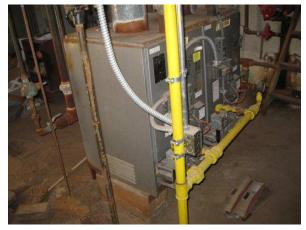
**Photo #4** View of Hydrotherm 400 MBH water tube hot water boiler in the boiler room.
