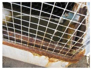
**Photo #2** View of some rusting that is occurring on the cooling tower around the basin.
