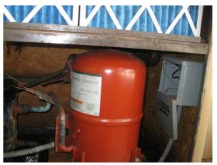
**Photo #9** View of compressor in the lobby area floor air handling unit.
