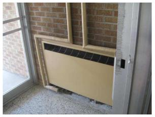
**Photo #13** View of hot water convection unit in one of the air locks for the station.
