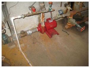
**Photo #3** View of condenser water pump that circulates condenser water from the cooling tower to the two floor air handling units in the station.
