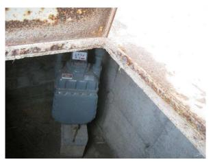
**Photo #17** View of 1000 CFH natural gas meter serving the building located in a pit on the south side of the station.
