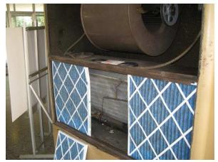
**Photo #8** View of the 1 HP fan in floor air handling unit with cover removed located in the main lobby.
