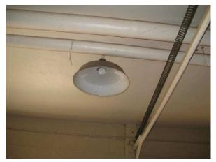
**Photo #29** View of incandescent fixtures in the baggage area of the station.
