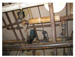
**Photo #6** View of one of the three control valves located on the ceiling of the boiler room.
