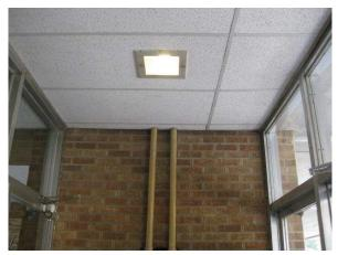
Photo #31 View of recessed lighting in the air lock.
