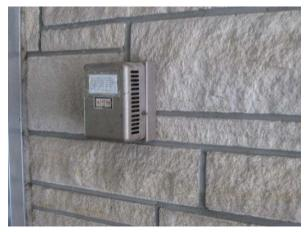
**Photo #16** View of older thermostat for one of the floor air handling units.
