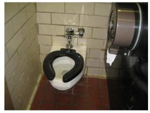
**Photo #22** View of typical wall hung water closet with flush valve in the restrooms.
