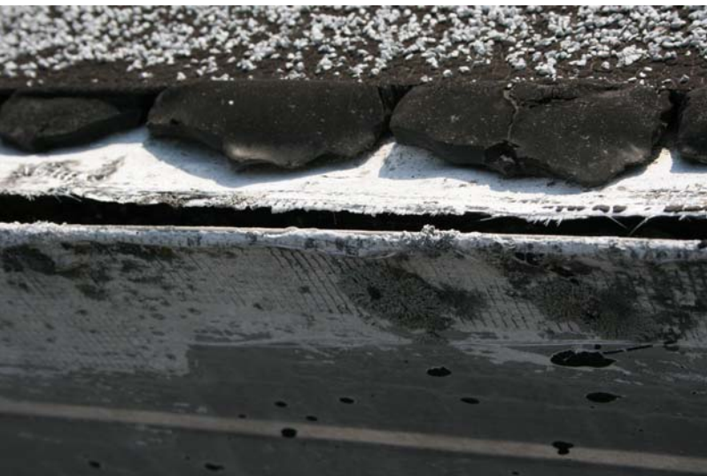
File Name : RoofEdgeSep.JPG Shooting Date/Time : 9/16/2009 11:44:44 AM
