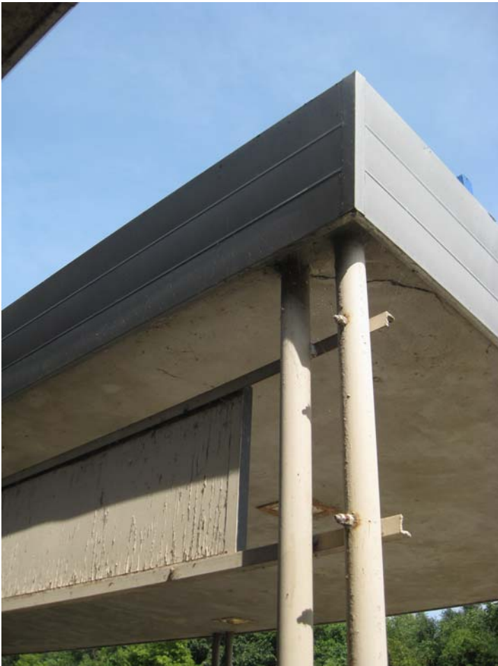
File Name : CanopyFascia.jpg Shooting Date/Time : 9/16/2009 1:03:06 PM
