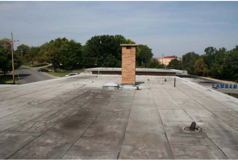
File Name : RoofLookingWest.JPG Shooting Date/Time : 9/16/2009 11:38:48 AM
