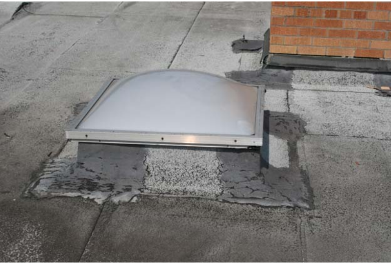
File Name : RoofSkylite.JPG Shooting Date/Time : 9/16/2009 11:34:44 AM
