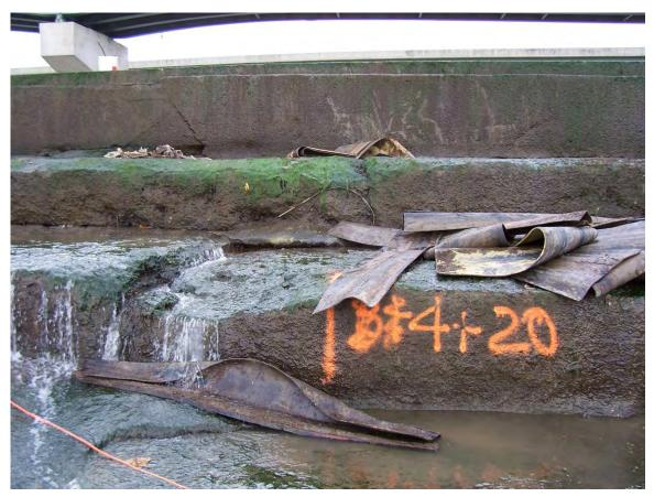
57. Sta 4+20. Severely deteriorated joint at top of bottom step. Seals from flashboards.
