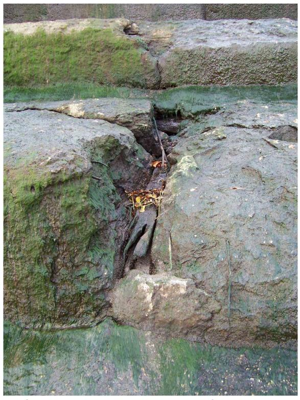
38. Sta 2+80±. Exposed timber and eroded concrete. Crack in bottom step.
