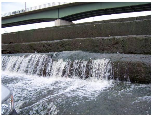
53. Sta 3+80±. Significant flow through Dam in numerous locations.
