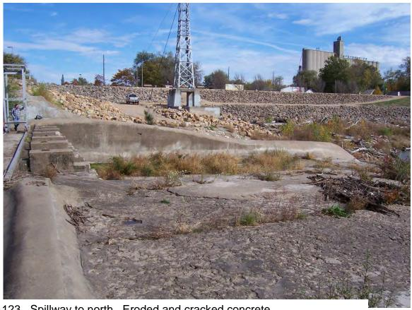
123. Spillway to north. Eroded and cracked concrete.
