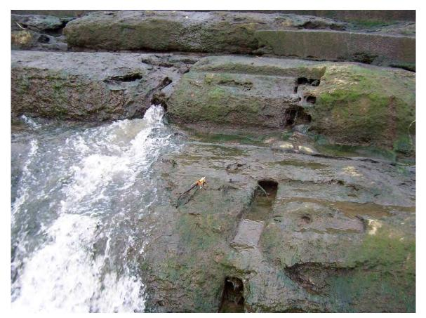
46. Sta 3+40. Eroded timber holes. Flow through timber hole. Severely deteriorated concrete.
