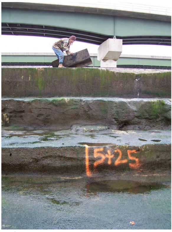
66. Sta 5+25. Exposed joints between first and second steps.
