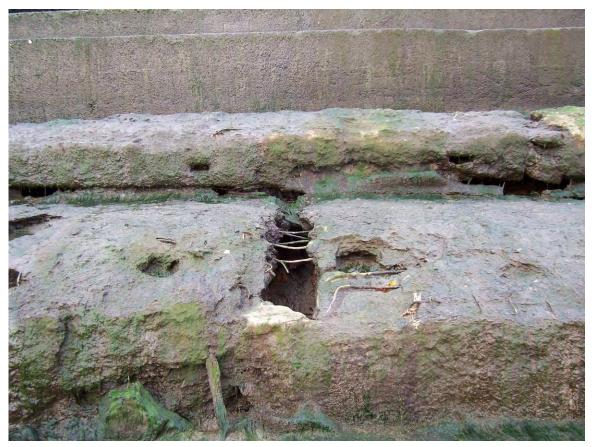
40. Sta 3+05. Eroded timber hole with exposed rebar. Exposed joint between steps.
