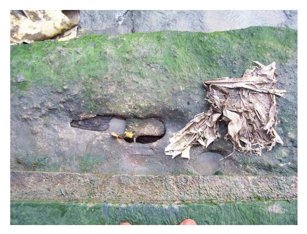
98. Sta 4+40±. Eroded concrete with exposed timber in top step.
