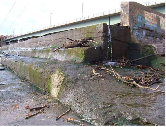
17. Sta 1+25. Eroded concrete at north end of dam.
