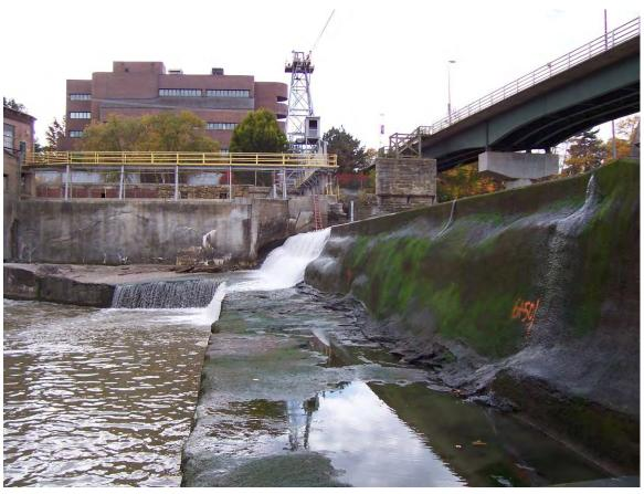
83. Sta 6+50 to south pneumatic flashboards. Eroded shotcrete.
