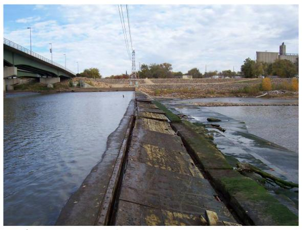
94. Sta 5+50 to north. Top of dam to south. Flashboards being repaired.
