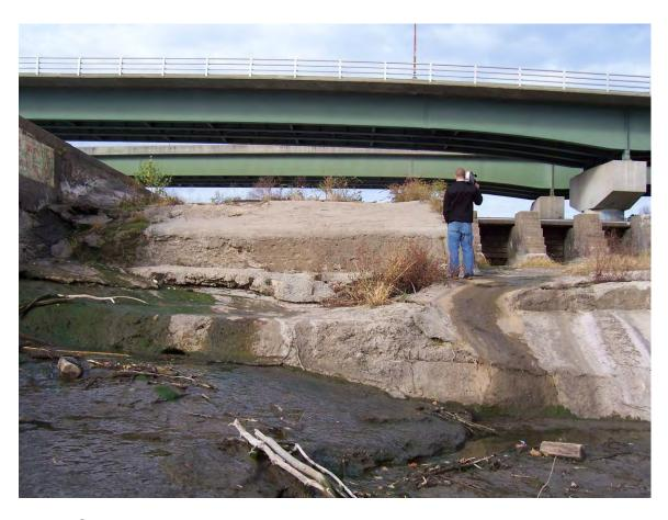
15. Sta 0+00. Eroded concrete and exposed joints in spillway.
