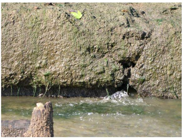
141. Sta 3+90±. Flow after grout bag repairs upstream.
