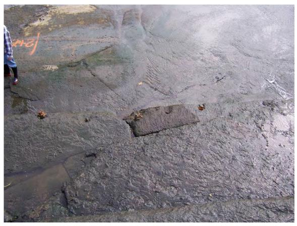
107. Sta 2+10 from top. Separated triangular section in bottom step.
