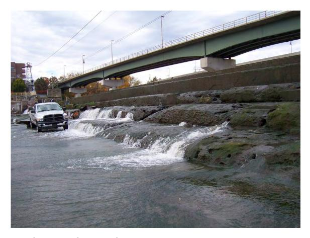
44. Sta 3+50 to Sta 3+90. Severely deteriorated steps. Flow through step joints and exposed, eroded timber holes. Large flow near Sta 3+90.
