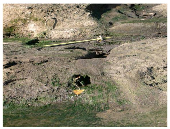
136. Sta 3+30. Exposed timbers between first and second steps. Severe deterioration of steps.
