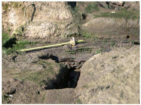
135. Sta 3+30. Exposed timbers between first and second steps. Severe deterioration of steps.
