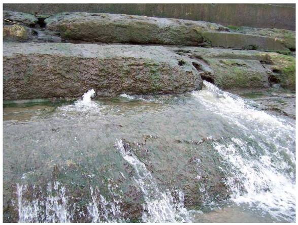
47. Sta  $3+45\pm$ . Eroded timber holes. Flow through timber hole. Severely deteriorated concrete.
