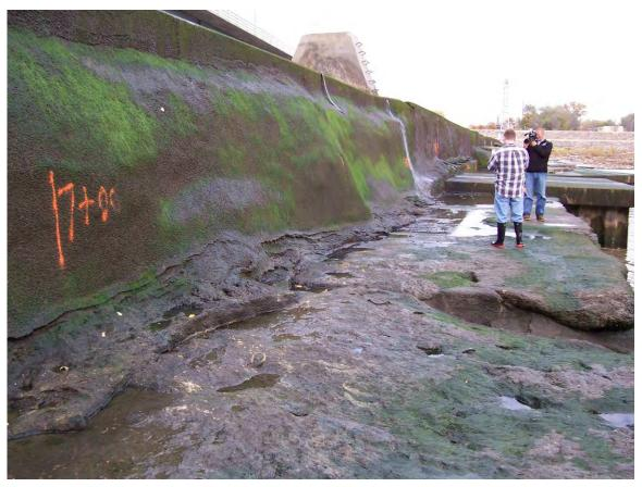
89. Sta 7+00 to north. Severely eroded apron and shotcrete.
