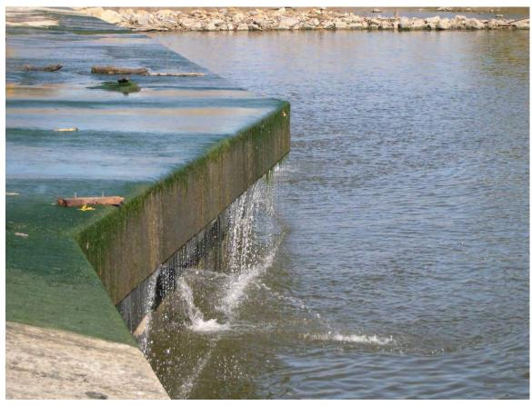
146. Sta 3+90±. Stream of flow through weep hole in piling below apron.
