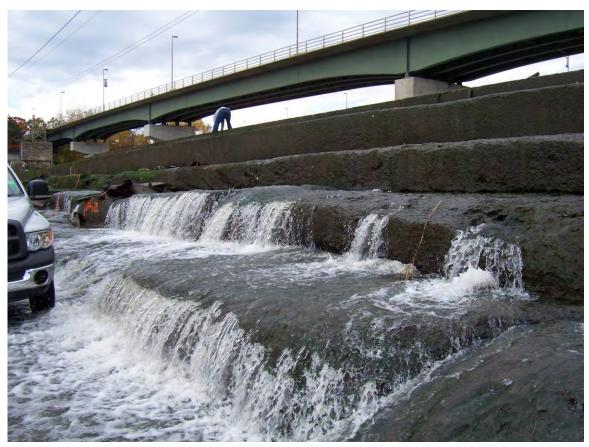
50. Sta 3+65 to Sta 4+20. Significant flow through dam in numerous locations.
