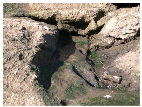
134. Sta 3+30. Exposed timbers between first and second steps. Severe deterioration of steps.
