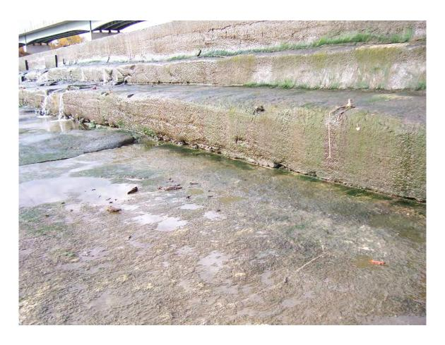
19. Sta 1+25 to 1+50. Exposed joints at bottom of dam steps. Eroded shotcrete at top step.
