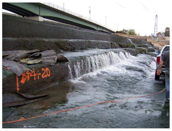
58. Sta 4+20 to North. Significant flow through dam.
