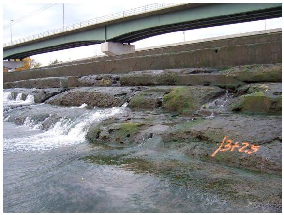
43. Sta 3+25 to Sta 3+50. Severely deteriorated steps. Flow through step joints and exposed, eroded timber holes.
