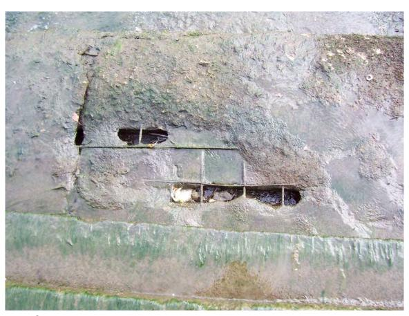
99. Sta 3+90±. Eroded concrete with exposed wire mesh in top step.
