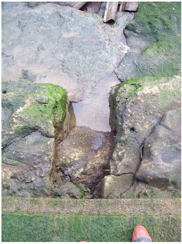
97. Sta 4+50 from above. Severe deterioration at old timber location. Multiple joints.
