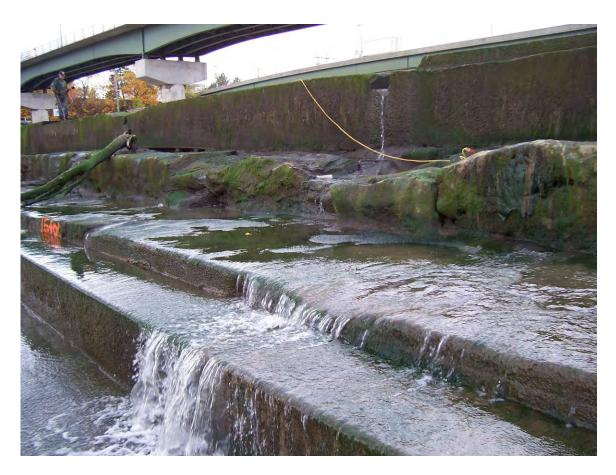
63. Sta 4+75 to 5+00. Severely eroded top step with flow through joint in step.
