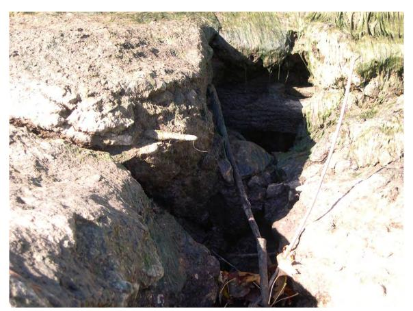
132. Sta 2+80. Exposed timber and eroded concrete. Crack in bottom step.
