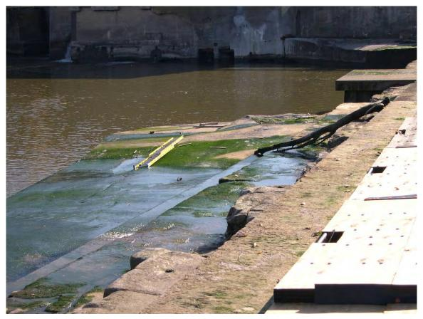
144. Sta 4+50±. Flow after grout bag repairs upstream.
