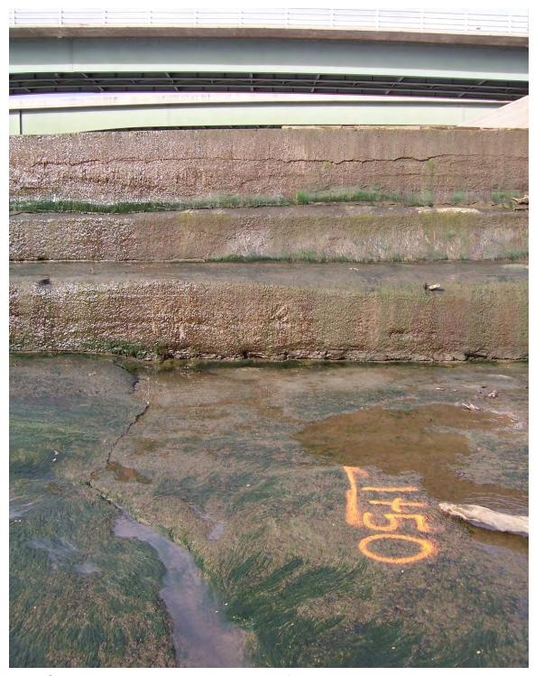
20. Sta 1+50. Exposed joints at bottom of dam steps – eroded shotcrete at top step. Exposed reinforcing rod in bottom step.
