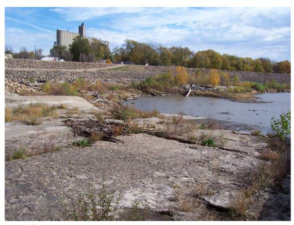
122. Spillway to northeast. Eroded and cracked concrete.
