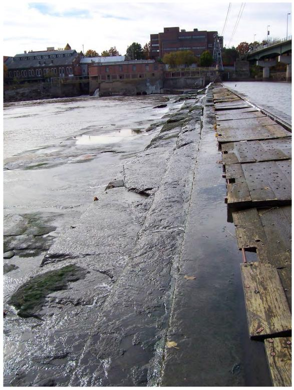
108. Sta 1+75 to south. Separated triangular section in bottom step. Eroded concrete steps.
