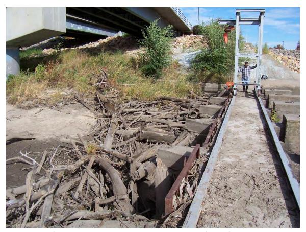
117. Top of spillway to north. Accumulated debris in front of gates.
