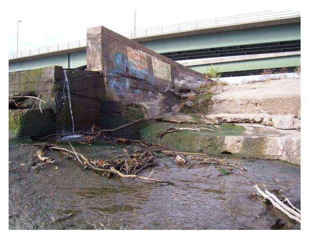
16. Sta 1+10. North wall of dam. Eroded concrete and exposed joints in spillway.
