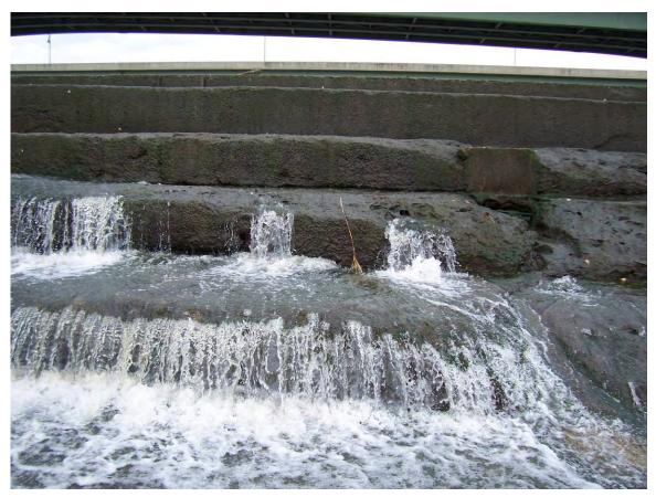
52. Sta 3+75±. Significant flow through Dam in numerous locations.
