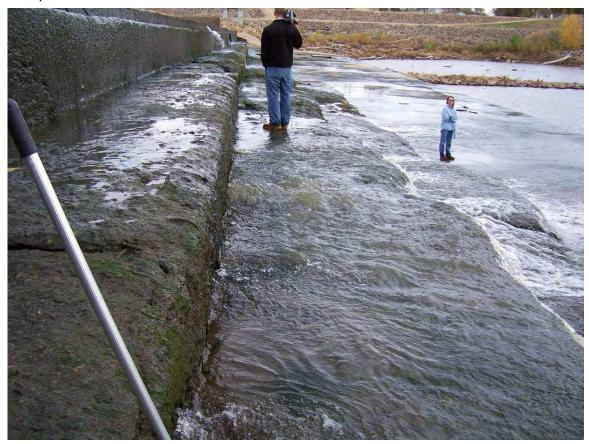
56. Sta  $3+90\pm$ . Looking north. Main flow point through dam. 4 ft deep hole at flow point.
