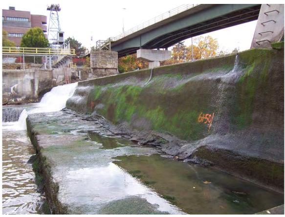
80. Sta6+50 to sour pneumatic flashboards. Eroded Shotcrete
