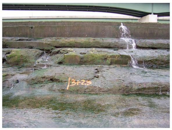
42. Sta 3+25. Severely deteriorated steps. Flow from channel at top of dam.
