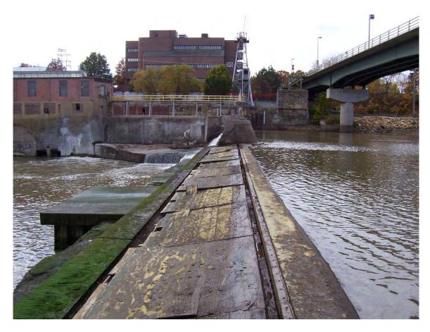
92. Sta 5+75. Top of dam to south. Flashboards being repaired.
