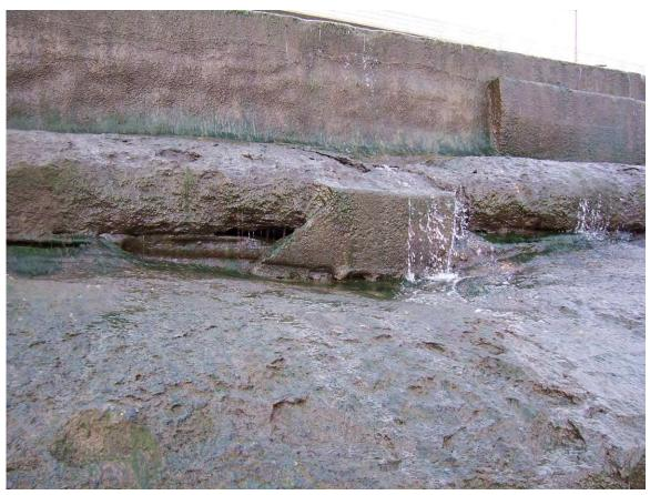
32. Sta 2+45. Deteriorated steps exposed joints.
