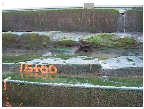
64. Sta 5+00. Deteriorated concrete at top step.
