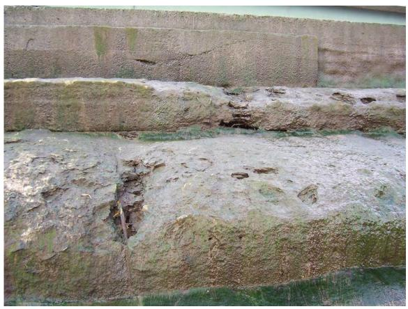
33. Sta 2+65±. Exposed timber holes and rebar. Eroded concrete. Exposed joint between steps.
