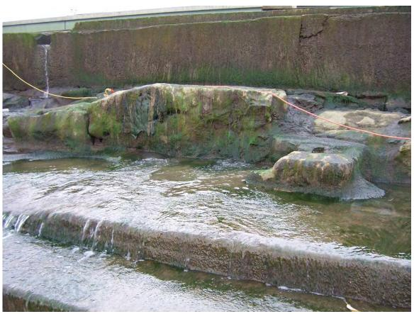
62. Sta 4+75±. Eroded and irregular steps with exposed joint and flow through joint.
