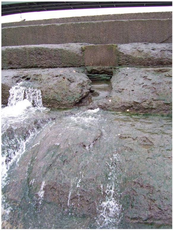
49. Sta 3+50. Eroded timber holes with flow through dam. Severely deteriorated steps.
