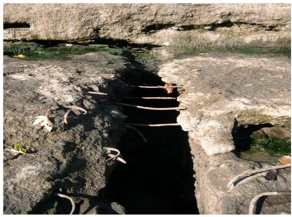
133. Sta 3+05. Eroded timber hole with exposed rebar. Exposed joint between steps.
