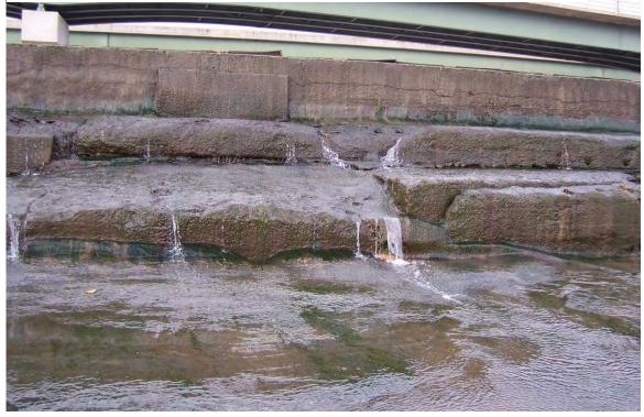
29. Sta 2+40±. Deteriorated steps. Exposed joints.
