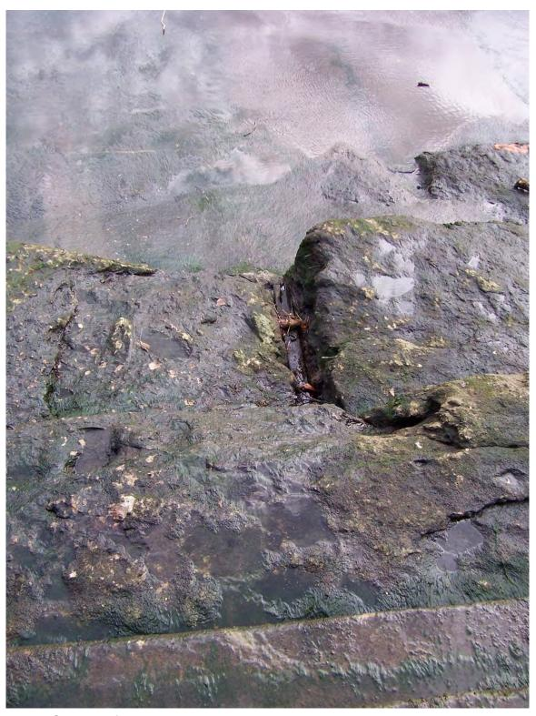
105. Sta 2+80 from top. Eroded timber and concrete.
