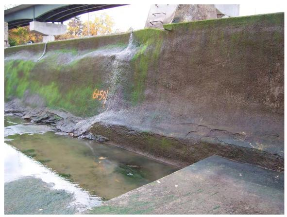
79. Sta 6+50 to south pneumatic flashboards. Eroded shotcrete.
