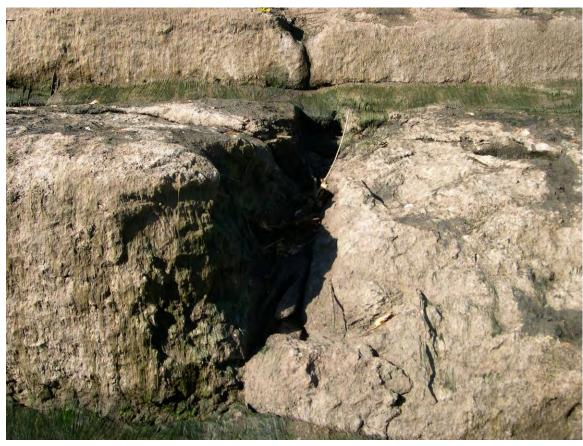
131. Sta 2+80. Exposed timber and eroded concrete. Crack in bottom step.
