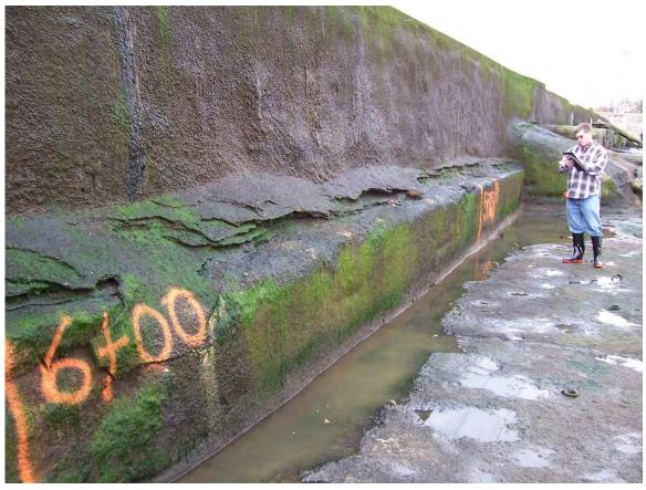
77. Sta 6+00 to 5+75 North. Eroded shotcrete.
