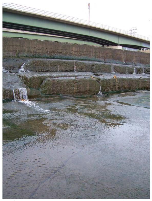
27. Sta 2+25±. Triangular section broken away in bottom step. Crack in apron that extends to edge of apron. Exposed joints between steps. Deteriorated steps.
