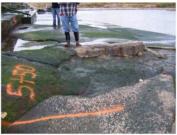
70. Sta 5+50. South end of steps. Exposed old sheet piling encased in apron. Eroded concrete with numerous exposed joints.
