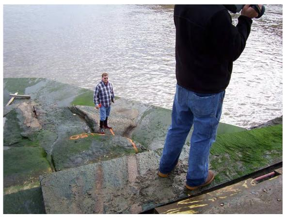
93. Sta 5+50. South end of steps. Eroded concrete with exposed joints.
