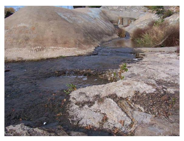
6. Sta 0+25±. Storm drainage flume north of spillway, eroded concrete
