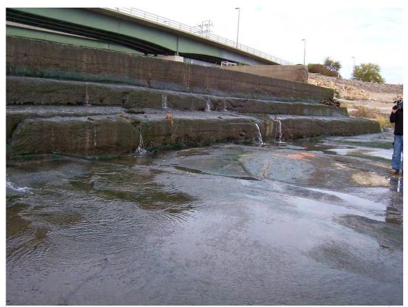
28. Sta 2+25. Back to Sta 2+00. Triangular section in bottom step. Crack in apron.
