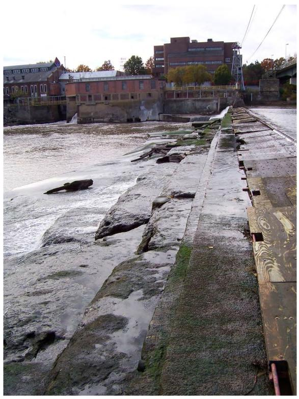
102. Sta 3+40 to south. Severe flow through dam. Cracked and deteriorated steps.
