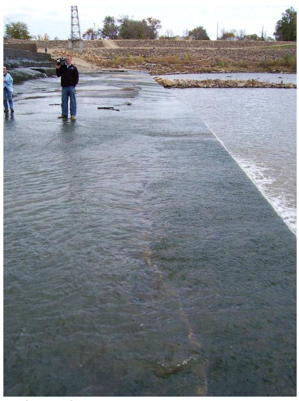
51. Sta 3+75±. Construction joint between old and new apron.
