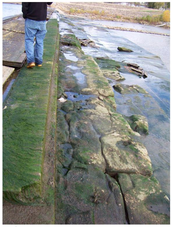
95. Sta 5+50 to 4+50 north. Eroded and uneven steps.
