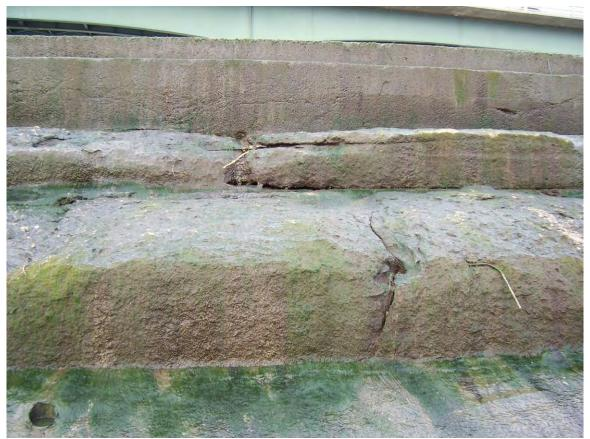
36. Sta 2+75±. Exposed joint and cracked middle step. Crack in bottom step. Weep hole.
