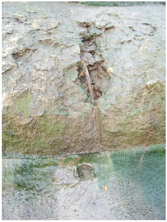
35. Sta 2+65. Exposed eroded timber at top of bottom step. Cast-In-Place weep hole at bottom of bottom step.
