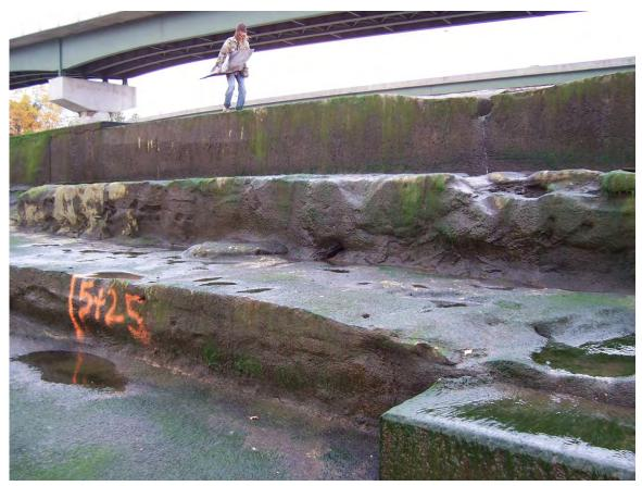
65. Sta 5+10 to Sta 5+25. Deteriorated concrete on top step. Exposed timber.
