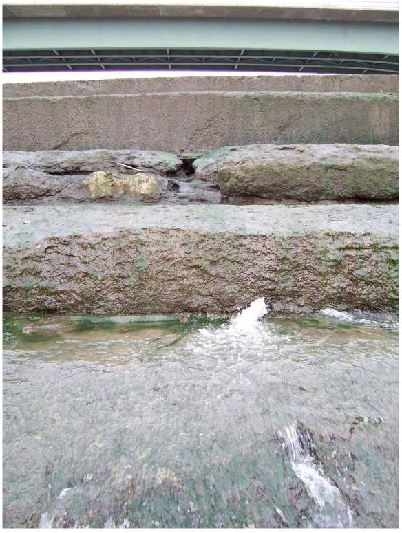
48. Sta 3+45±. Eroded timber hole and crack in top step. Flow through joint between 1<sup>st</sup> and 2<sup>nd</sup> step.
