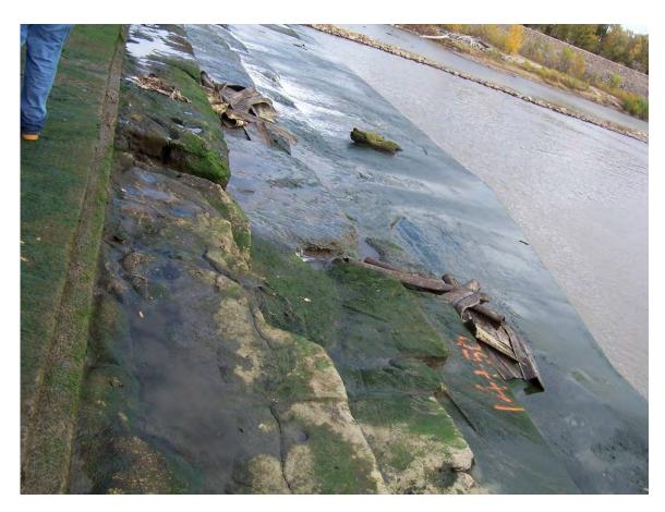
96. Sta 4+50. Eroded and cracked steps.
