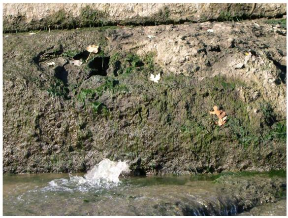
139. Sta 3+55. Flow after grout bag repairs upstream.
