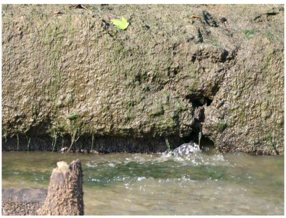
140. Sta 3+80. Flow after grout bag repairs upstream.
