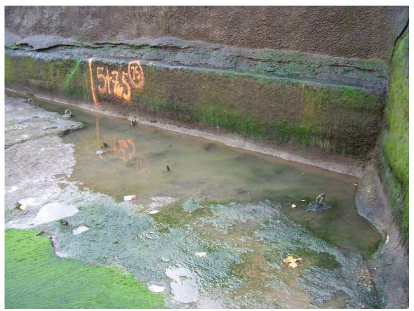
72. Sta 5+75. Eroded shotcrete. Depression with exposed spikes and tie-rings.
