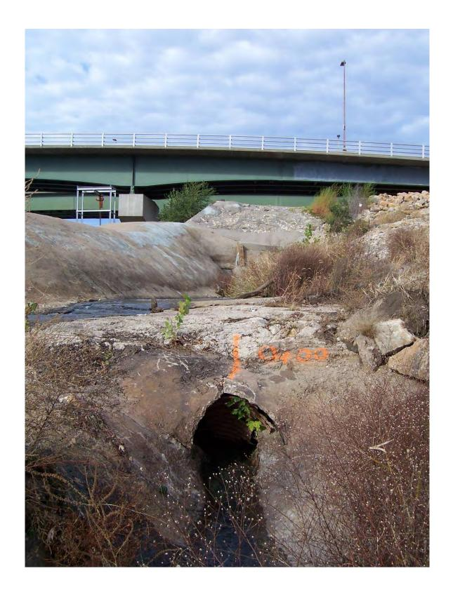
1. Station 0+00, North end of dam, storm drain, deteriorated concrete along storm drainage flume
