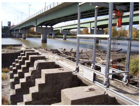
115. North end of spillway, accumulated debris ahead of spillway inlet.
