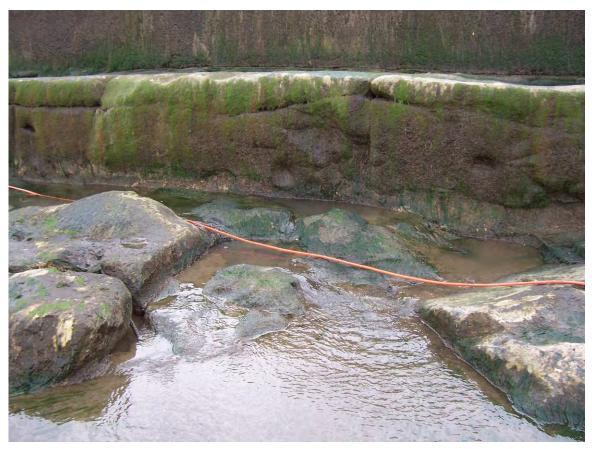
61. Sta 4+50±. Severely eroded concrete and exposed boulders.
