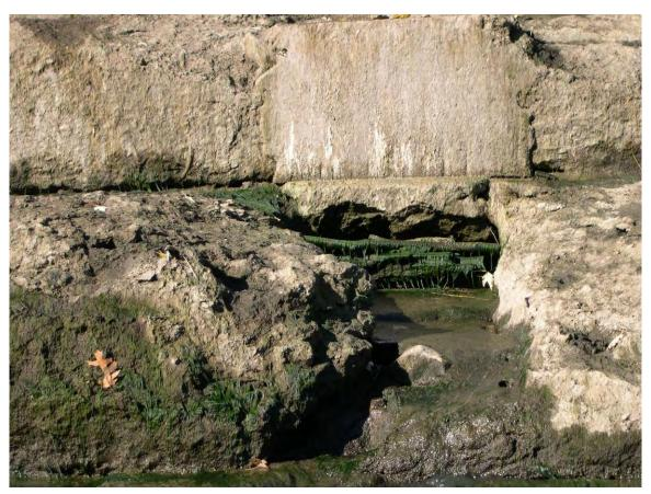
138. Sta 3+50. Eroded timber holes with flow through dam. Severely deteriorated steps.
