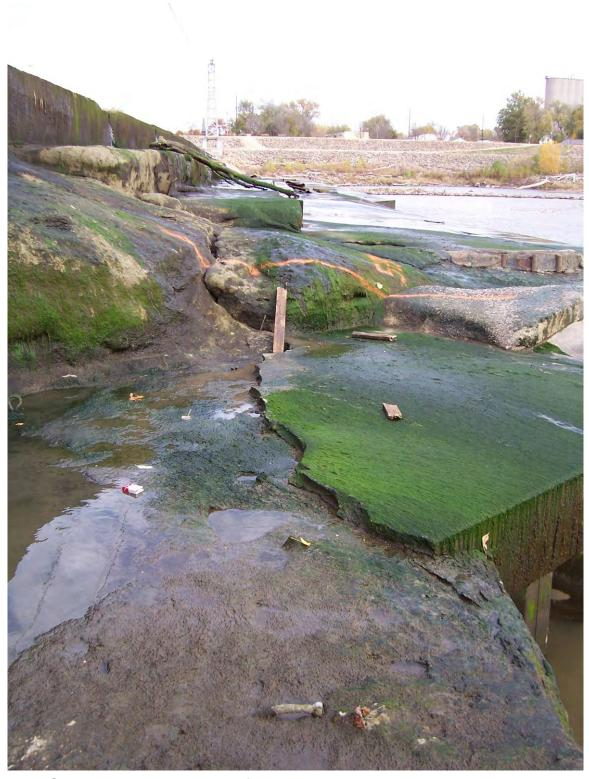
90. Sta 5+60. Eroded portion of new apron. Exposed spike in old apron.
