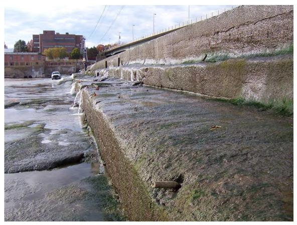
21. Sta 1+50 to Sta 2+00. Eroded concrete steps and shotcrete. Exposed reinforcing bar.
