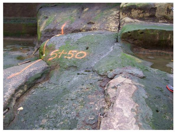
69. Sta 5+50. South end of steps. Eroded concrete exposed joints.
