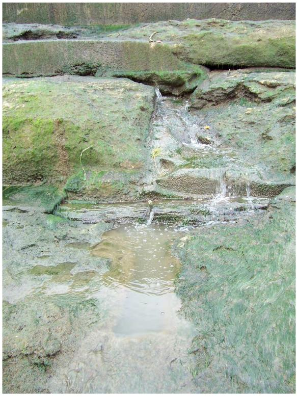
45. Sta 3+30. Exposed timbers between first and second steps. Severe deterioration of steps.
