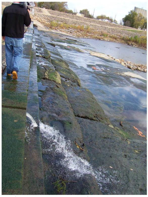
103. Sta 3+00 from top. Flow over dam top. Severe step deterioration.
