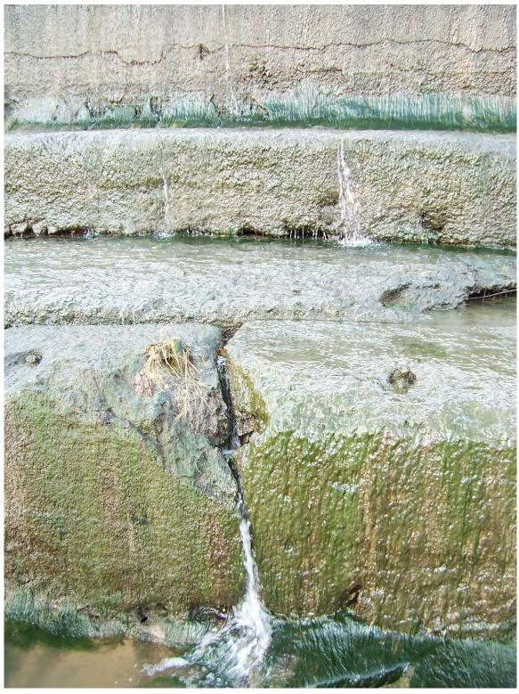
26. Sta 2+10. Crack in lower step. Exposed joint between steps. Eroded shotcrete with exposed wire mesh. Triangular crack beginning.
