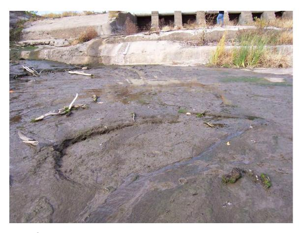
14. Sta 0+75. Eroded concrete in spillway.
