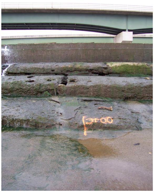
39. Sta 3+00. Exposed and eroded timbers exposed rebar. Severely deteriorated bottom steps.
