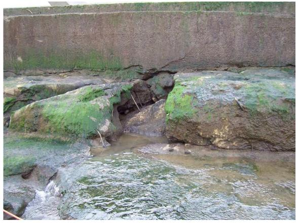
59. Sta 4+40±. Severely deteriorated steps. Exposed joints between steps.
