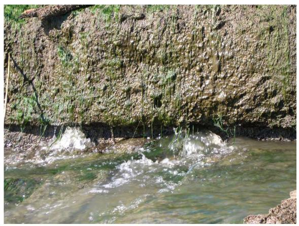
142. Sta 3+90. Flow after grout bag repairs upstream.
