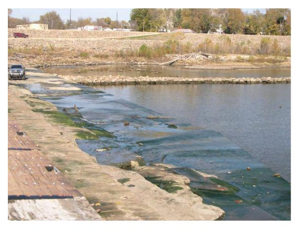
145. Sta 3+90±. Flows after grout bag repairs upstream.
