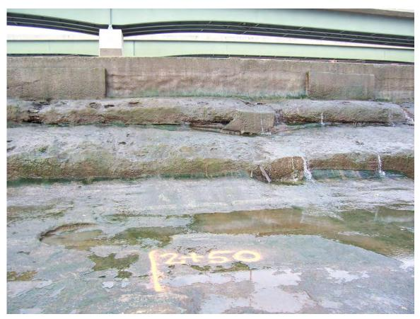
30. Sta 2+50. Exposed joints between steps. Eroded concrete in top step. Exposed rebar at old timbers.
