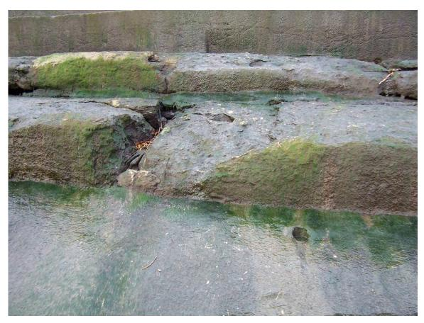
37. Sta 2+80±. Exposed timber and eroded concrete. Crack in bottom step.
