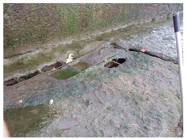
55. Sta 3+90±. Severely deteriorated concrete with exposed rebar in top step.
