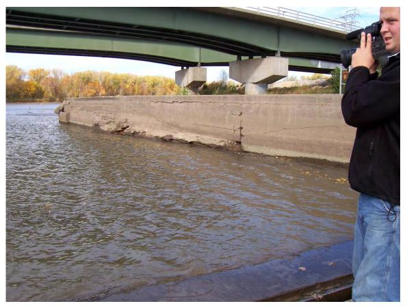
109. Sta 1+75 top of dam to north dam wall. Eroded concrete and open joints.
