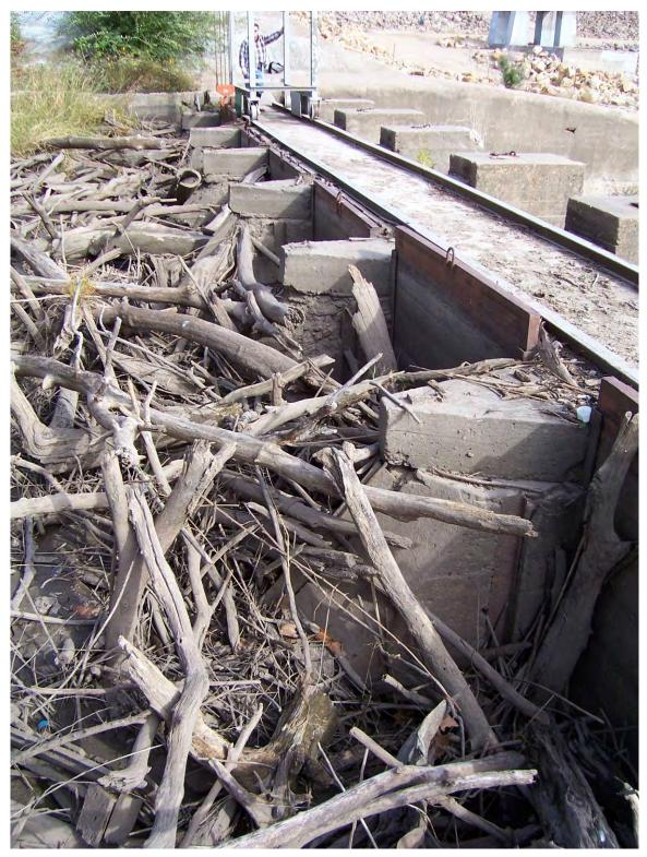
126. Accumulated debris in front of spillway gates.
