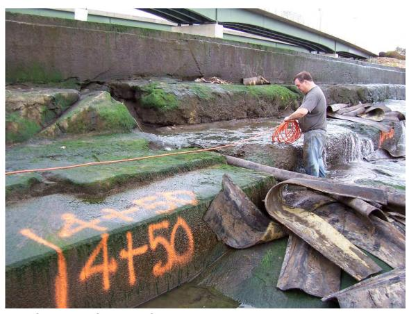
60. Sta 4+50 to Sta 4+40. Severely deteriorated steps. Exposed joints between steps.
