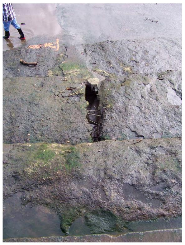
104. Sta 3+00 from top. Eroded timber hole with exposed rebar.
