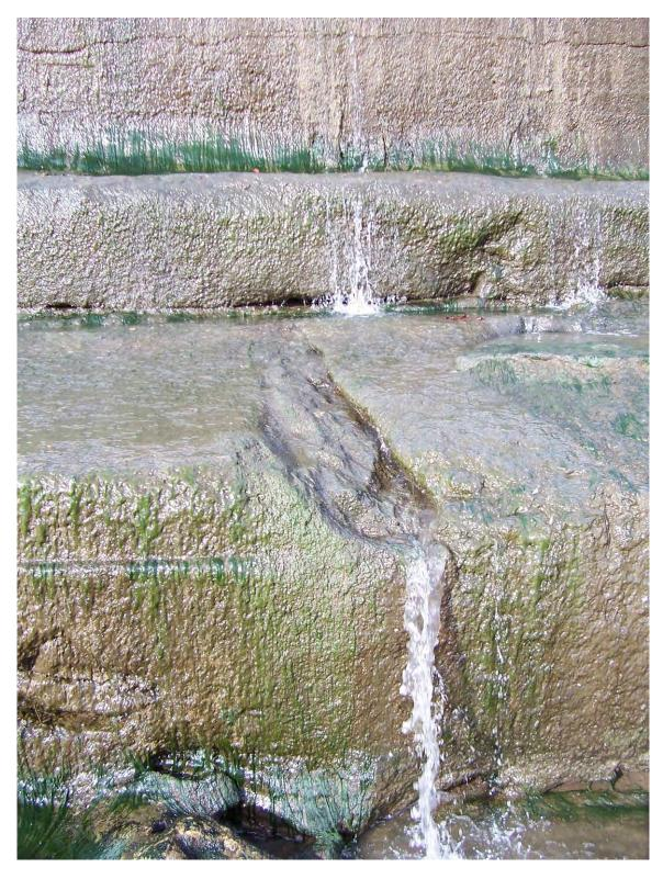
23. Sta 1+80. Eroded concrete on bottom step. Exposed joints between steps. Eroded shotcrete on top step.
